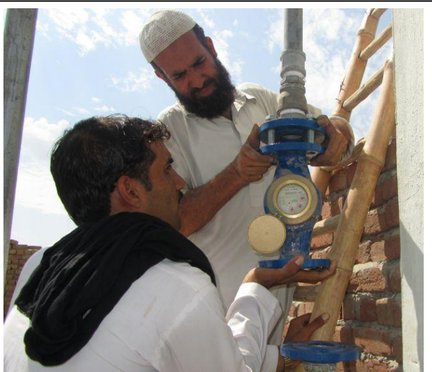
Figure 9 Installation of Flow Meter
